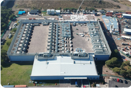
Eastern Creek Surfside Data Centre Buildings 2,3 & 4
