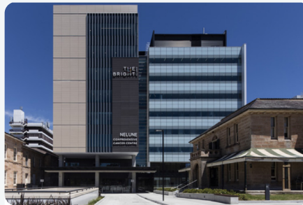
The Bright Alliance Building – Prince Of Wales Cancer Centre
